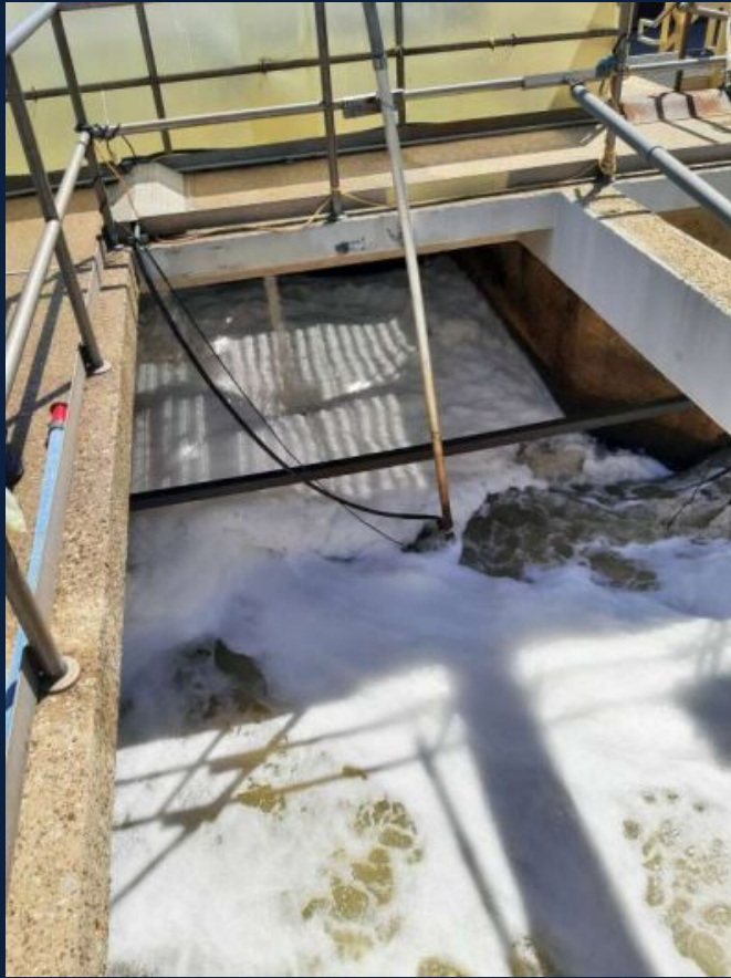
Final discharge with persistent foam/scum/solids, final effluent sample with amber color.
