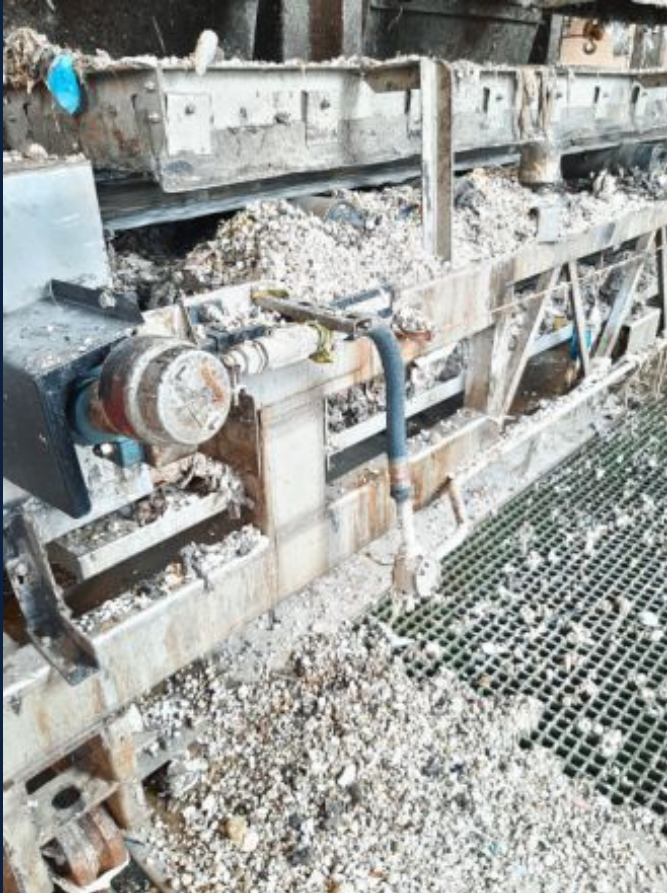
“Trash” clogging conveyor belts
